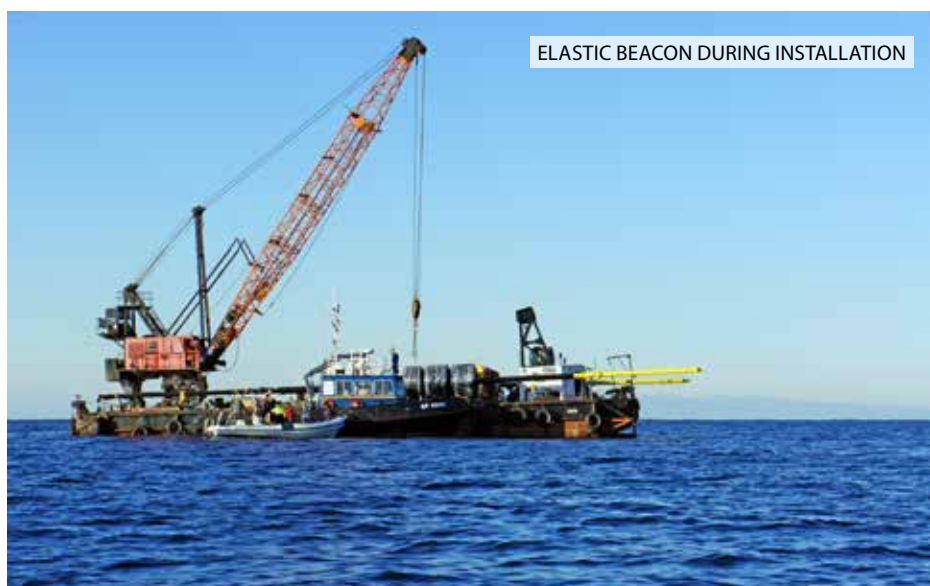
ELASTIC BEACON DURING INSTALLATION
