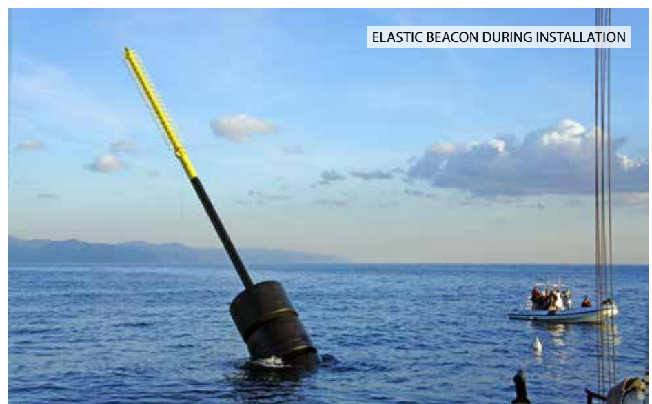
ELASTIC BEACON DURING INSTALLATION
