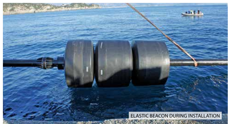
ELASTIC BEACON DURING INSTALLATION
